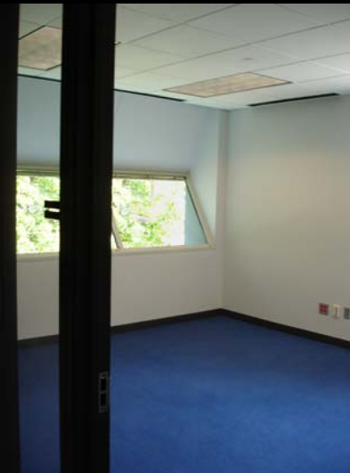
A special thickened wall design employed tipped glazing to shy away from the summer sun angle but bounced in the light to naturally brighten the perimeter offices.
