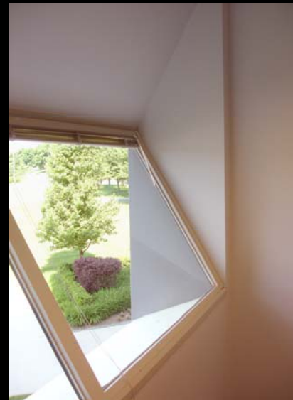
A special thickened wall design employed tipped glazing to shy away from the summer sun angle but bounced in the light to naturally brighten the perimeter offices.
